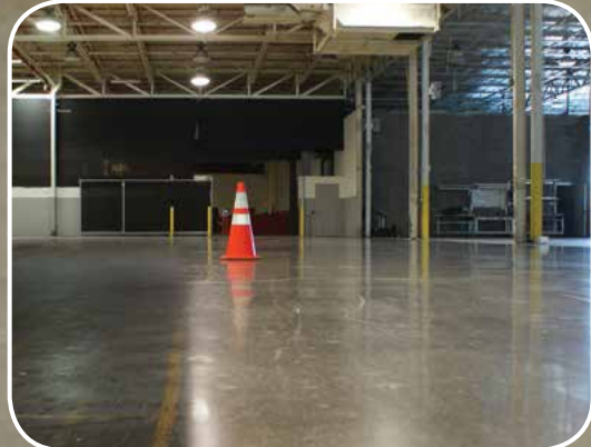
CONCRETE POLISHING
